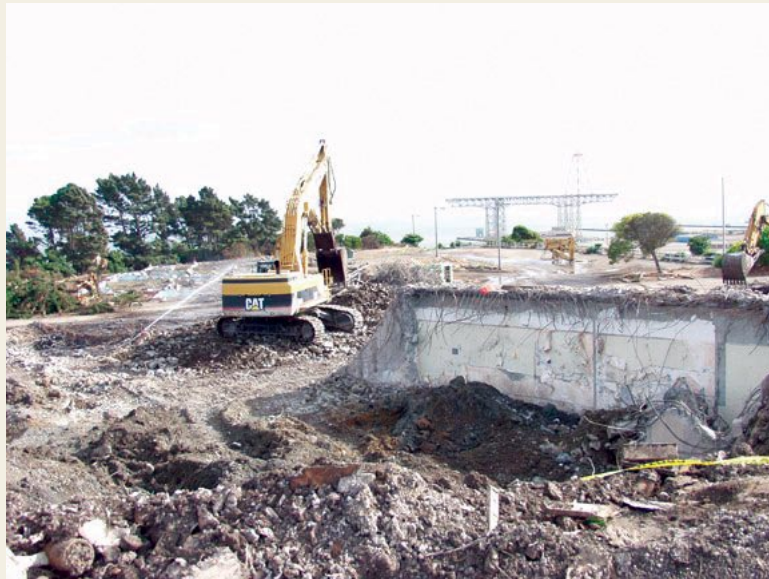
Construction continues on the Hilltop portion of Parcel A
